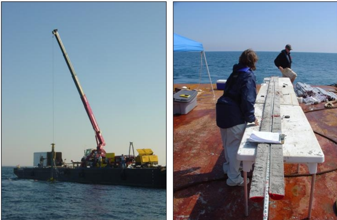
Figure 11. Crane deployment of the 271B Alpine Pneumatic vibracore system (left). Vibracore logging being conducted aboard the work barge during the vibracore operations (right).
